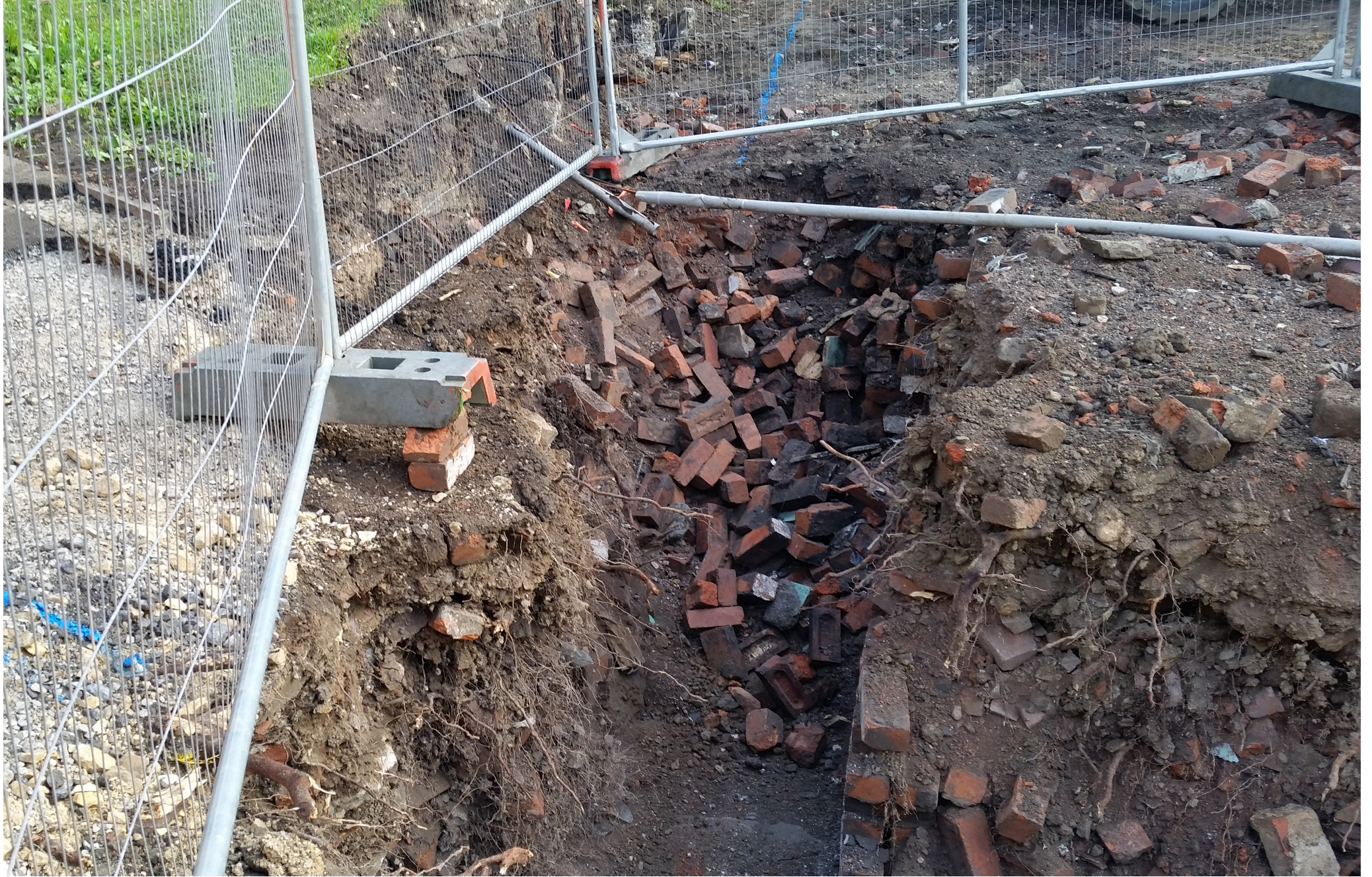
Uncover redbrick basements
