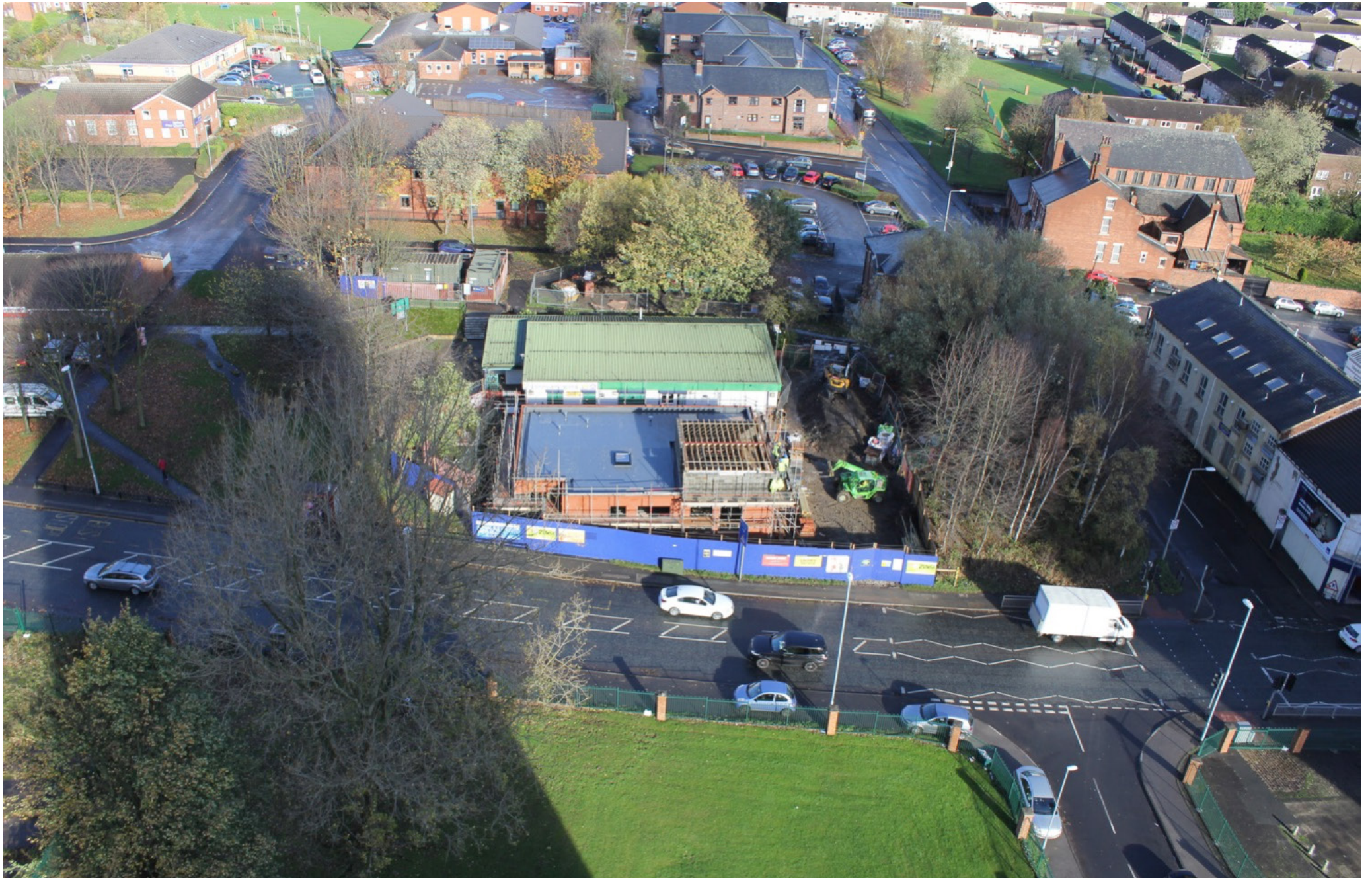
Construction view from neighbouring tower
