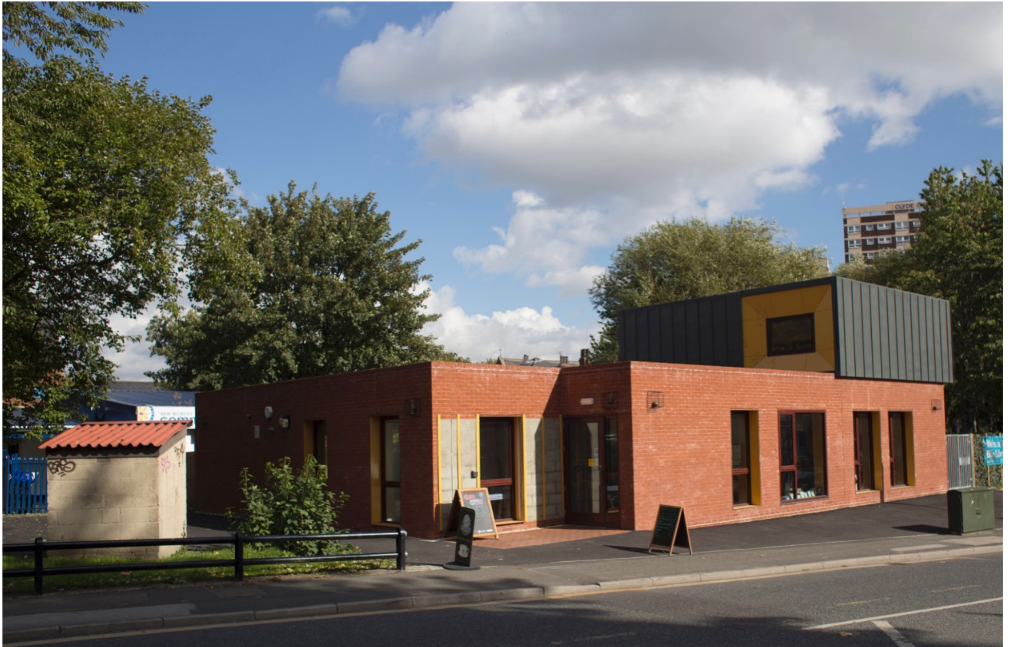
View from Tong Rd - awaiting entrance panels
