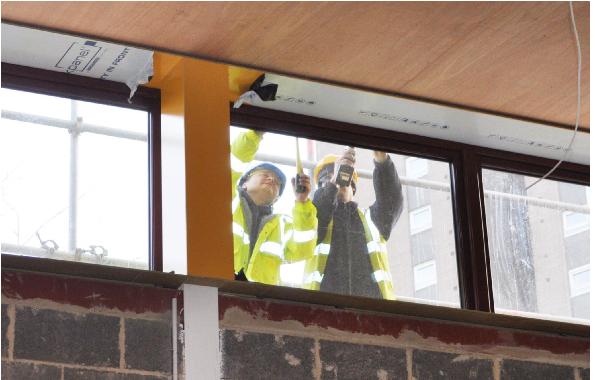
Install windows and doors
