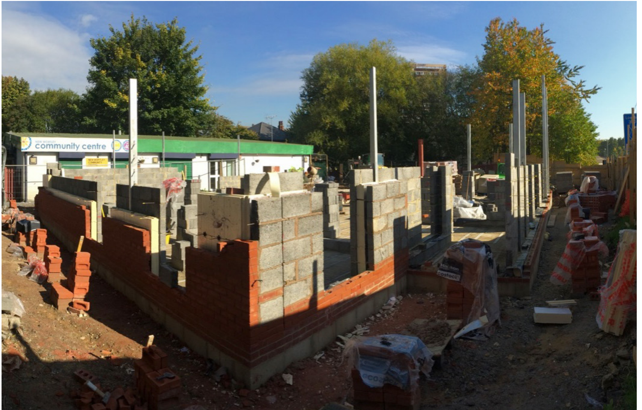
Brick & block walls
