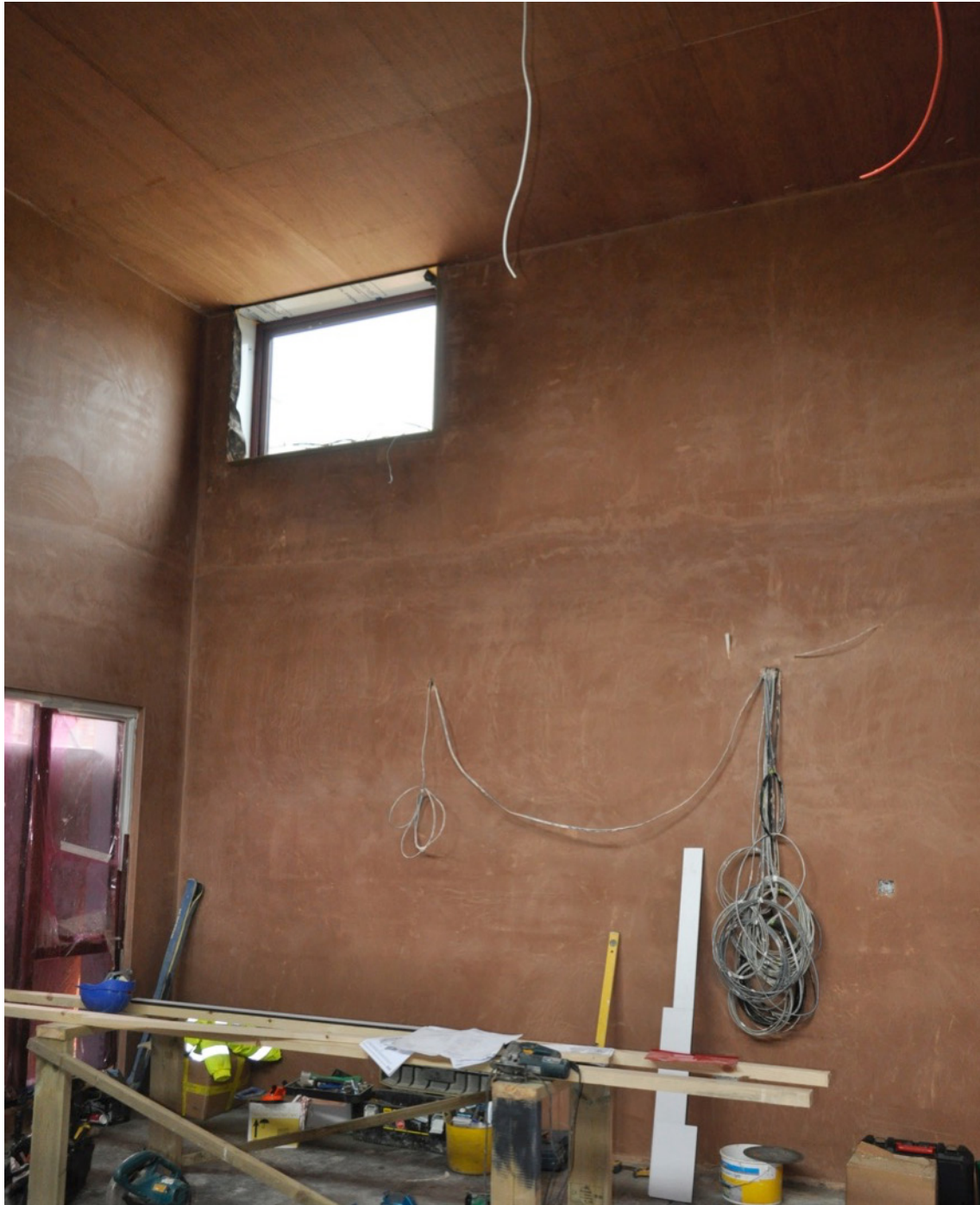
Plaster internal walls
