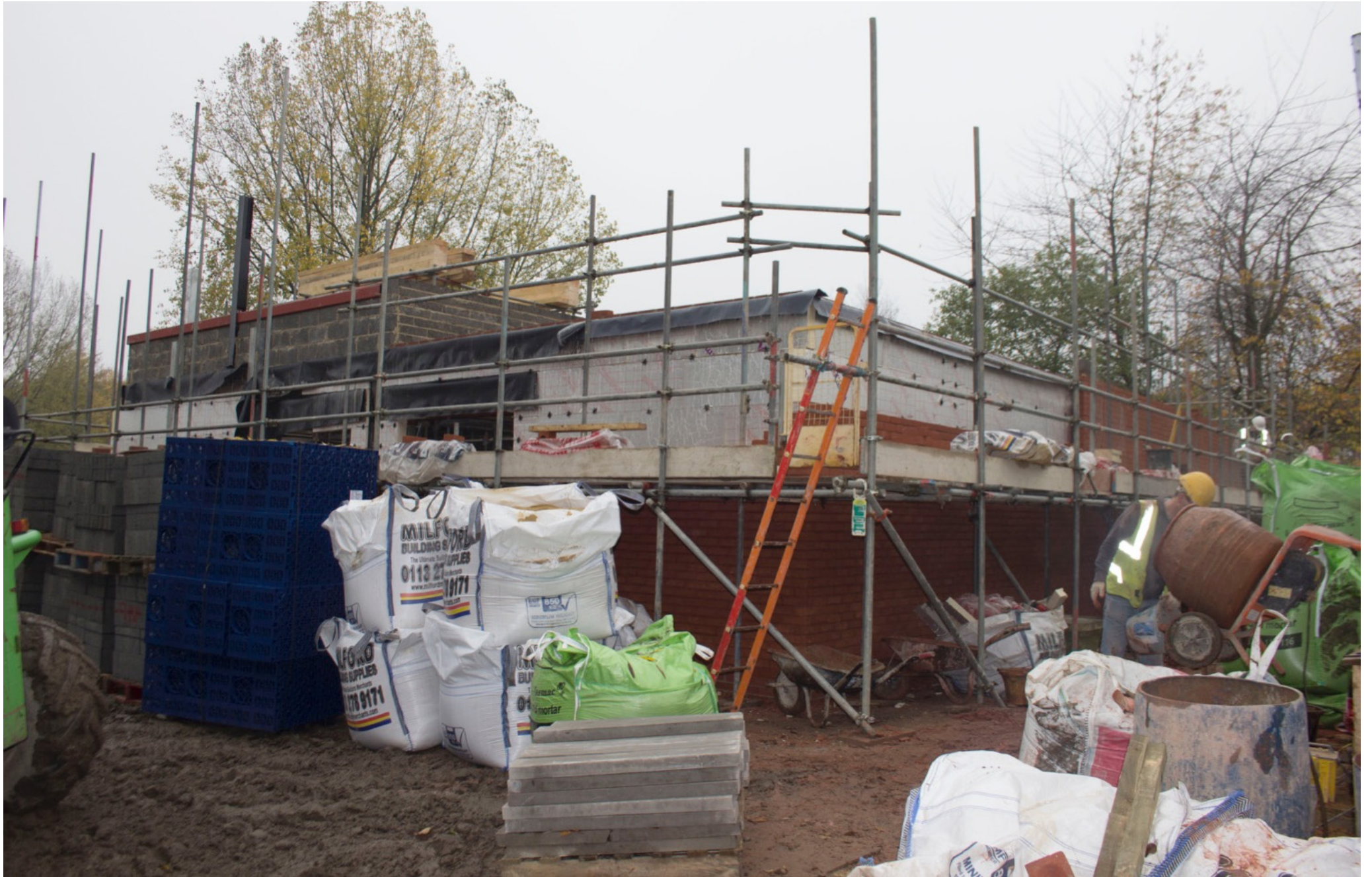
Brick & block walls
