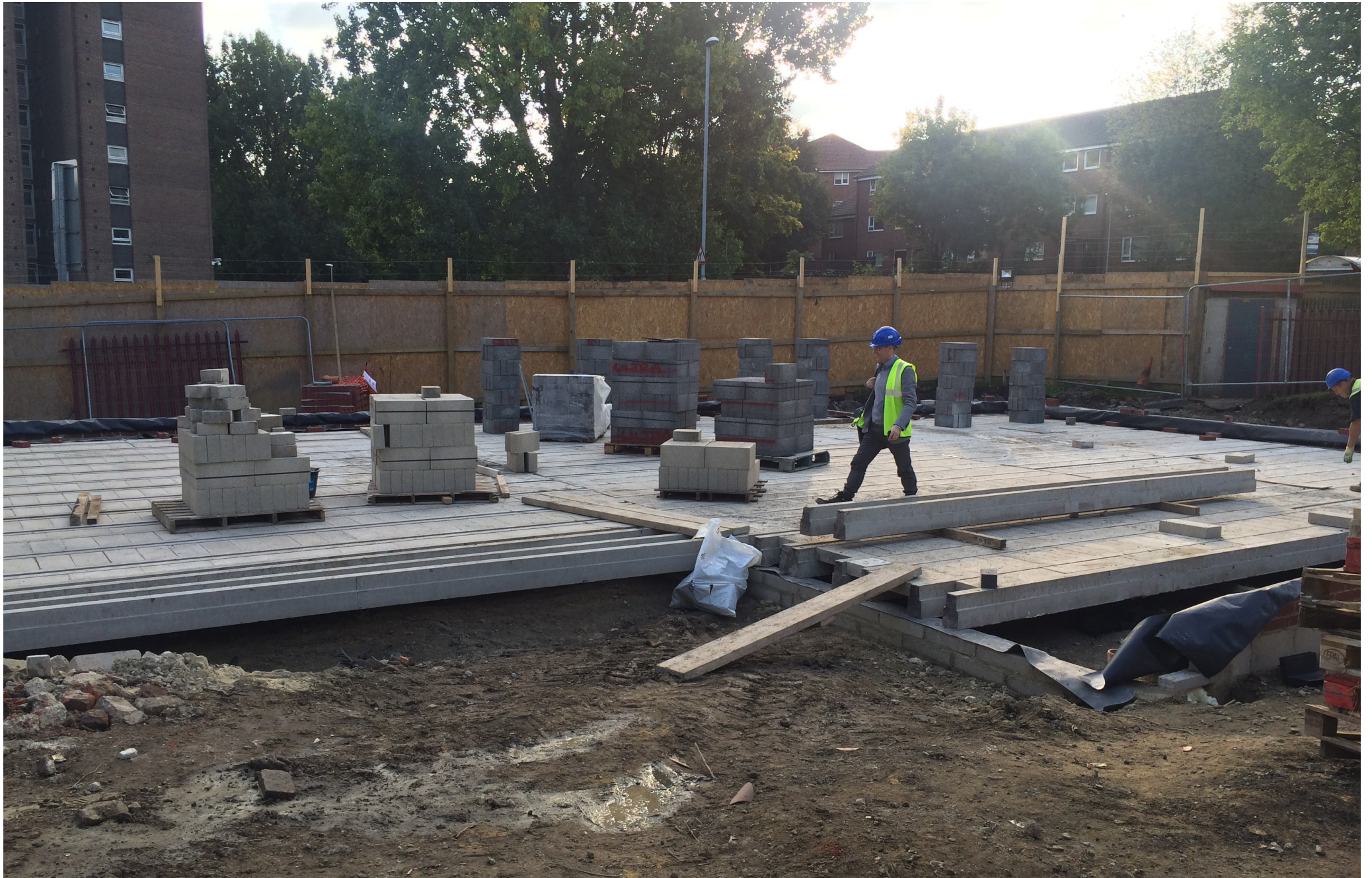
Beam & Block floor
