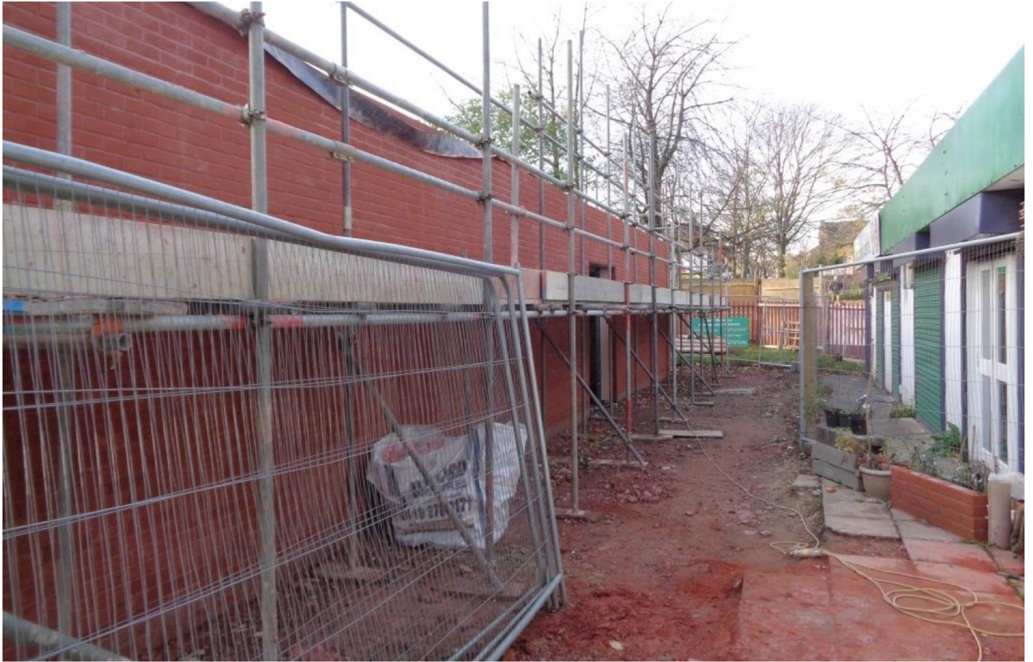
Brick & block walls
